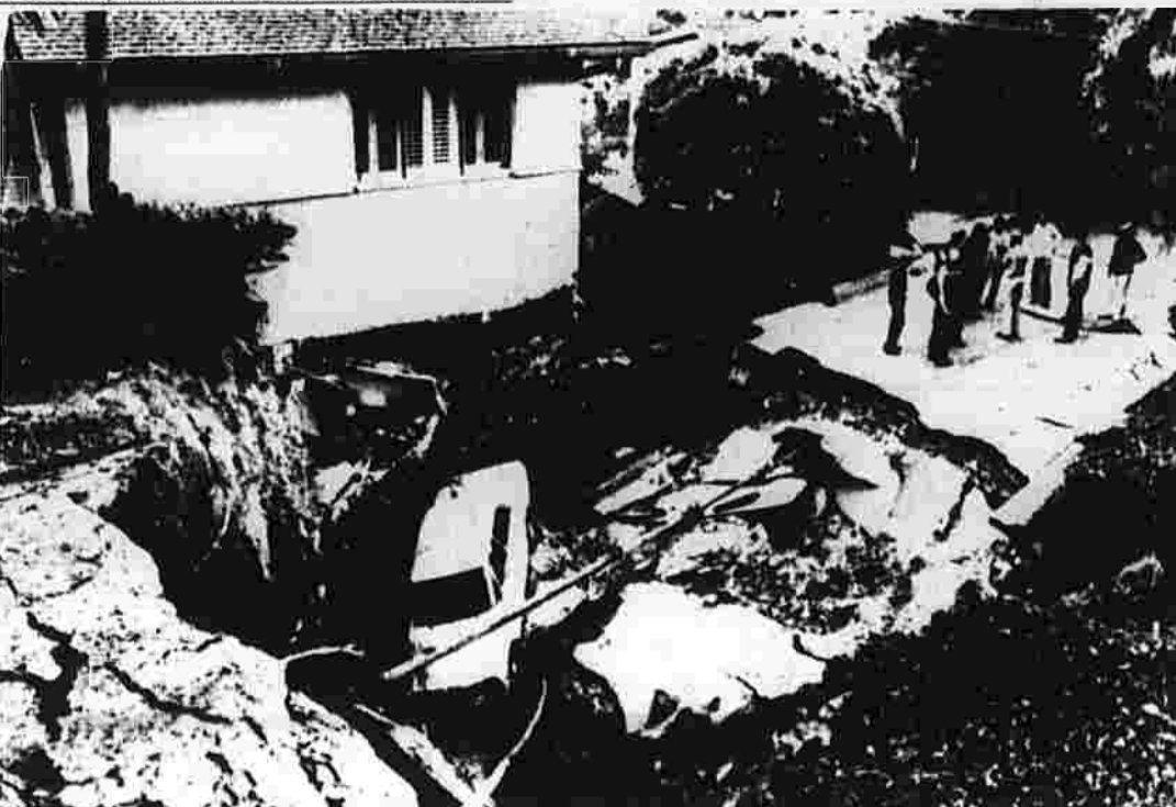
Police and rescue teams stand near a 40-foot fissure that undermined house on left and swallowed up car. More than 40 homes were damaged or demolished in the slide, forcing the evacuation of 260 persons. Damage is expected to exceed $2 million. (UPI photo)
